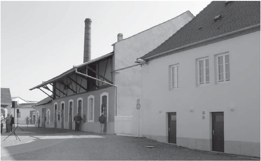
The stables (rear) now a store
